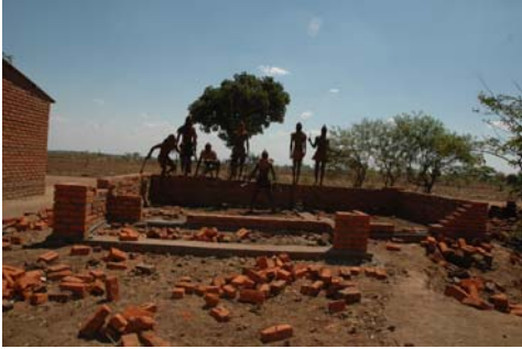
Foundations to kitchen/store
